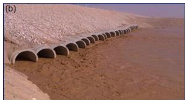
Photo 1. (a & b) Under desert road culverts carried out in the western Assiut City desert.
