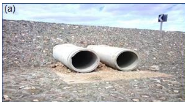
Photo 1. (a & b) Under desert road culverts carried out in the western Assiut City desert.
