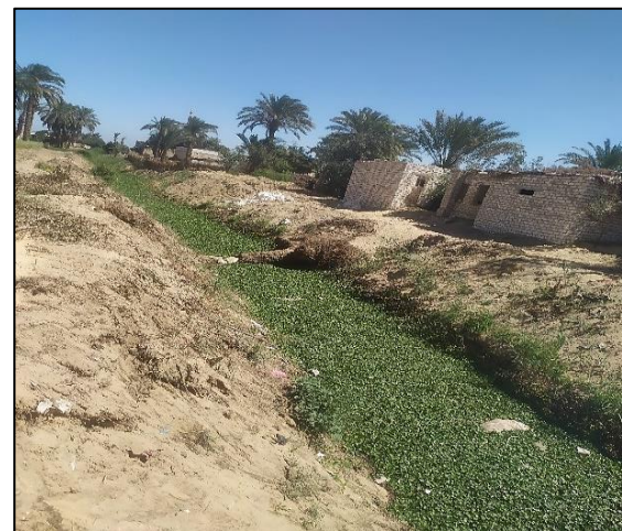
Photo (2): Unlined canal section
