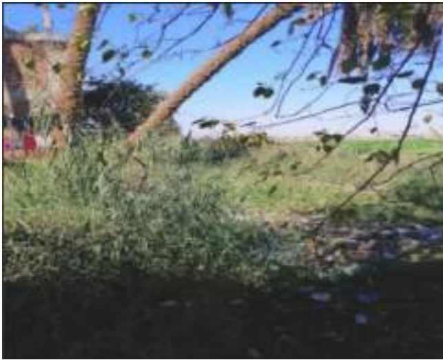
Fig. 10. Weeds block the stream of Bani Mohamed canal.
