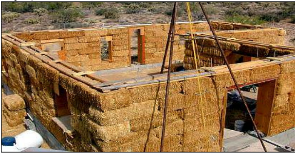
Figure 5: Load bearing structure
