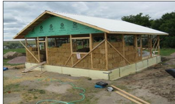
Figure 7: Non-load bearing structure
