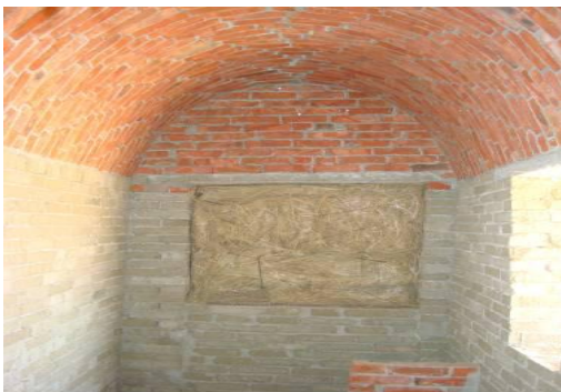
Figure 11: The vault by R-brick and red- brick
