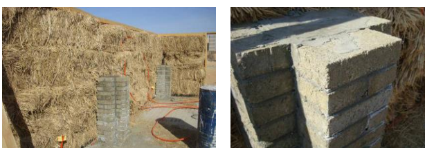
Figure 12: The 6 corner made of R-bricks
