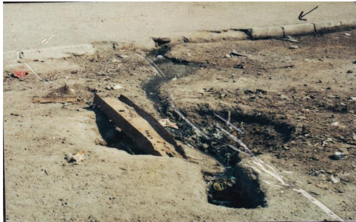
Fig (5) : A course for the discharge of domestic uses water in one of the districts of Basra city in the inspection basin of storm sewer ending in Khadek branch. 8/11/2015
